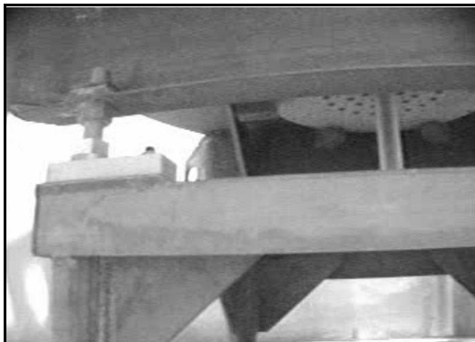
Figure 6. View of the reactor structure.
